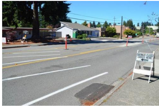
Figure 49. Temporary mid-block crosswalk with ramp. Note: non-compliant MUTCD sign on barricade. Source: myedmondsnews.com
