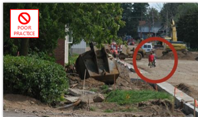
Figure 3. Children bicycling in active work area.
