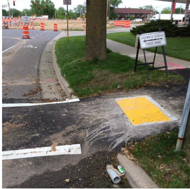
Figure 6. Tactile warning with contrasting color at temporary curb ramp in work zone. Source: UW-TOPS Lab
