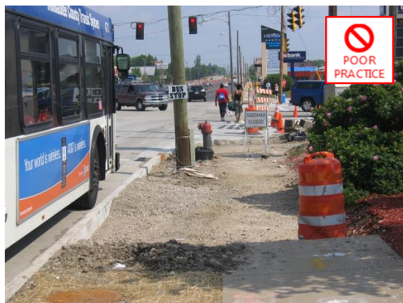
Figure 70. Passengers discharged into sidewalk closure.
