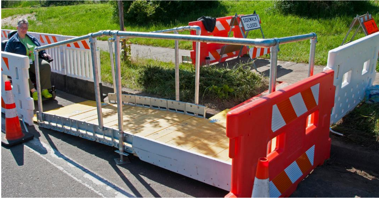
Figure 5. Temporary Pedestrian Ramp. Source: Oregon DOT
