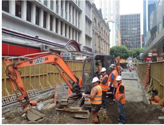
Figure 53. Temporary plywood walls.
