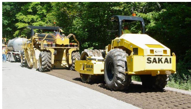
Figure 77. Full-depth stabilized soil reclamation equipment. Source: roadrecycling.org/FDR-Process
