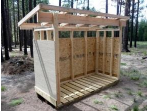
Figure 72. A temporary bus shelter constructed with lumber and plywood. Source: flickr.com
