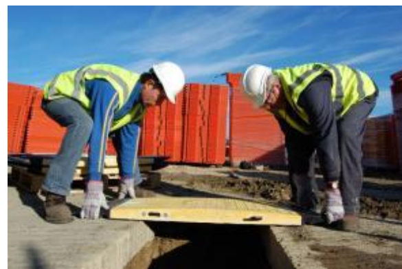
Figure 44. Modular trench cover system to accommodate varying length of open trench.
