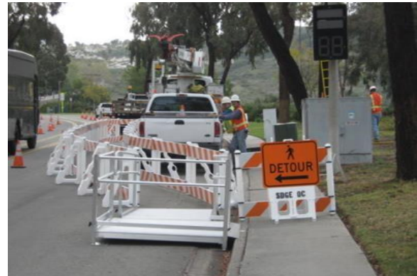
Figure 20. Pedestrians temporarily rerouted around work area.
