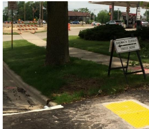
Figure 24. Pedestrians routed around closed sidewalk at intersection work area with ADA compliant temporary crosswalk. Note: detectable barrier needed at end of sidewalk instead of Type III barricade.
