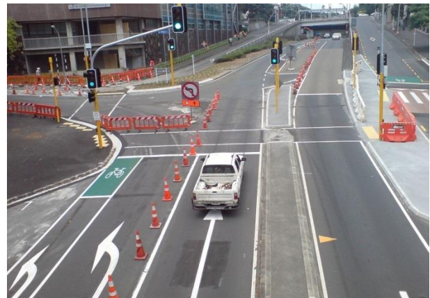
Figure 84. Thoughtful staging provides safe pedestrian and bicycle access during construction (Australian example).
