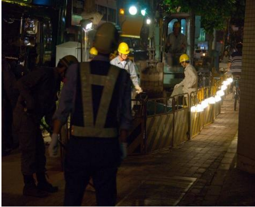
Figure 67. Temporary lighting mounted on barricades.
