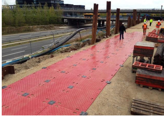
Figure 78. Pedestrian matting application Source: Oxford Plastics LLC
