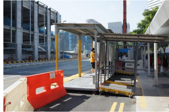
Figure 73. Temporary bus shelter constructed mainly from scaffolding materials. Note: ADA ramp used, but ADA detectable edge needed at end of platform. Source: photobucket.com
