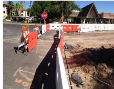
Figure 57. ADA compliant longitudinal pedestrian barricade for channelizing pedestrians away from traffic and work areas.
