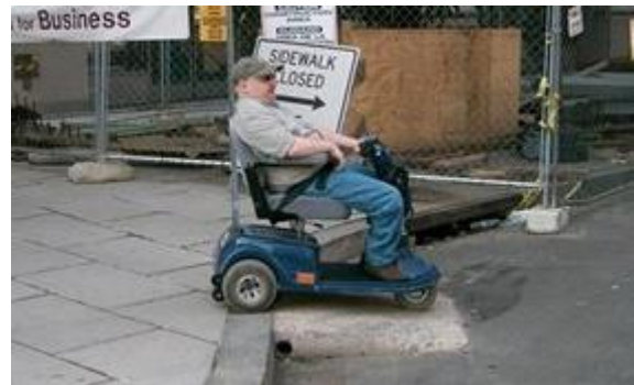
Figure 38. Temporary curb ramp (concrete). Source: Photo reproduced with the permission of the American Traffic Safety Services Association (ATSSA)
