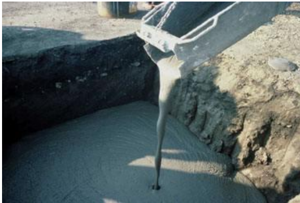
Figure 75. Controlled Low Strength Material (CLSM) discharging from mixer truck. Source: FHWA /pavement/recycling
