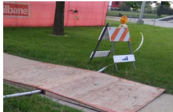
Figure 35. Water hose protected by double ramp allowing pedestrians to safely cross hose.
