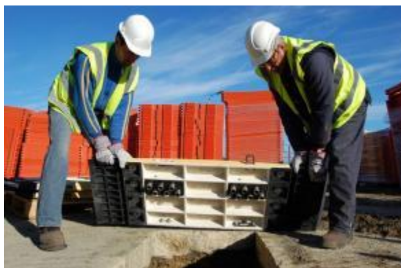
Figure 43. Modular road and sidewalk trench cover system with self-pinning anchors and sloping edges.
