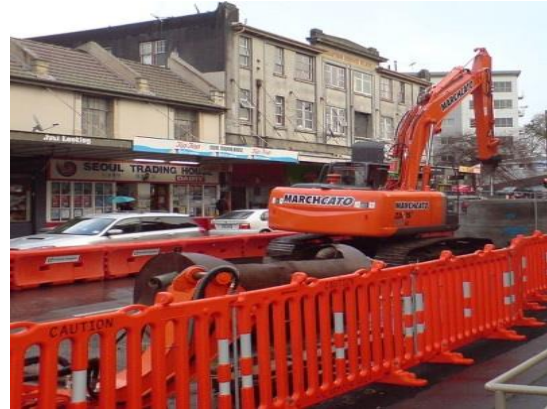
Figure 28. Well-delineated work activity area.
