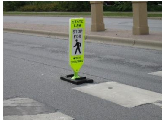
Figure 51. Vehicular signage for temporary crossing. Note: non-MUTCD compliant sign legend.
