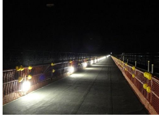
Figure 68. Temporary lighting mounted on fences. Note: ADA detection rail correctly used on right side fence.
