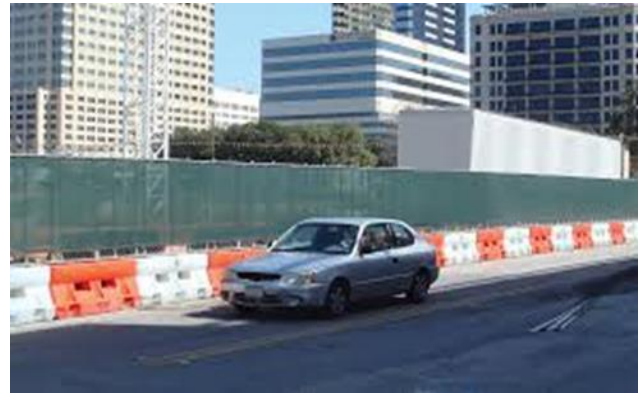
Figure 55. Water filled longitudinal channelizer barricade system used to support visual screening fence next to a work site.
