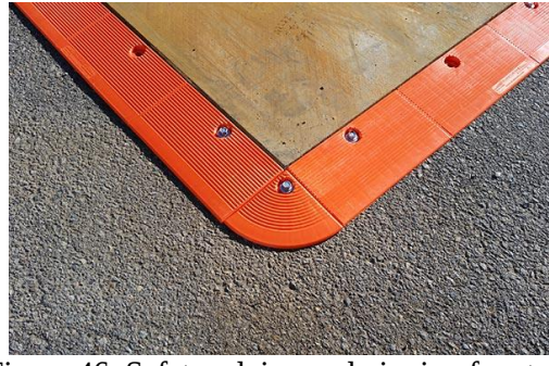
Figure 46. Safety edging and pinning for steel plates. Source: Platelocks.com
