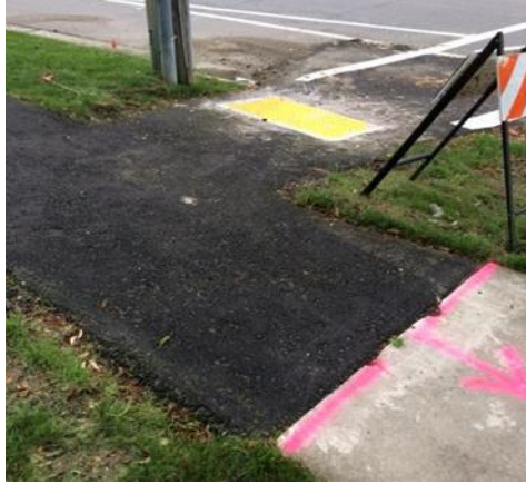
Figure 2. Temporary ADA pedestrian crossing Source: UW-TOPS Lab
