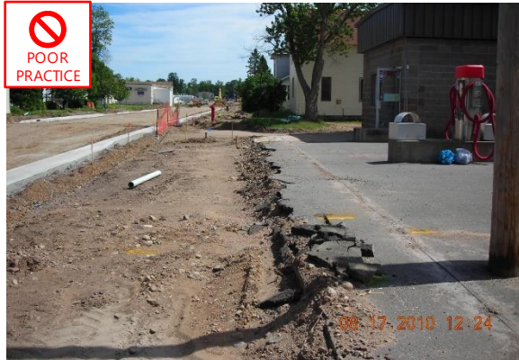
Figure 19. Complete removal of all pedestrian pathways.
