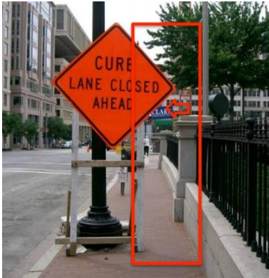
Figure 14. Pedestrian hazard due to low sign. Note: Non-MUTCD compliant uniform font on sign.
