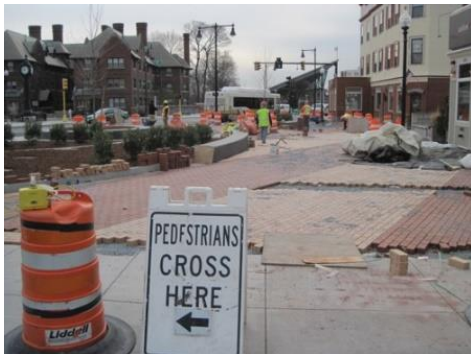
Figure 50. Pedestrian signage for temporary crossing. Note: Work area requires full pedestrian closure and compliant MUTCD regulatory pedestrian sign, i.e. MUTCD R9-11a.
