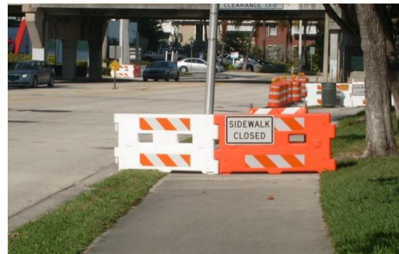
Figure 26. Sidewalk terminus fully barricaded.
