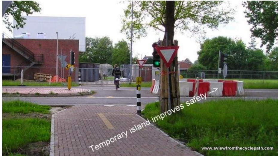
Figure 17. Temporary traffic island allowing two-stage bicyclist crossing of a busy roadway (Dutch example).
