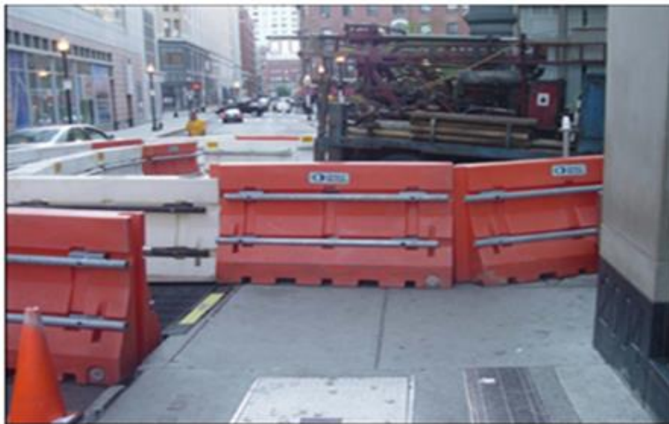
Figure 4. Work area with controlled pedestrian access.
