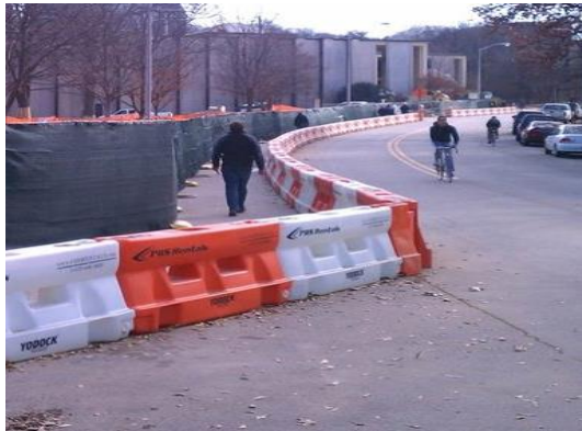
Figure 54. Longitudinal channelizer barricade system defines effective unobstructed pathway for pedestrians.
