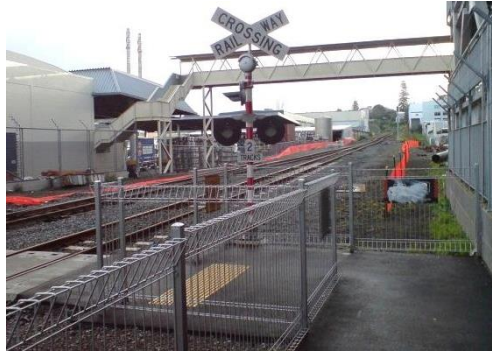
Figure 74. Temporary pedestrian rail line crossing. (UK example, non-MUTCD compliant RR x-buck) Source: Wikimedia/Level_Crossing_At_Kingdon_Street_West
