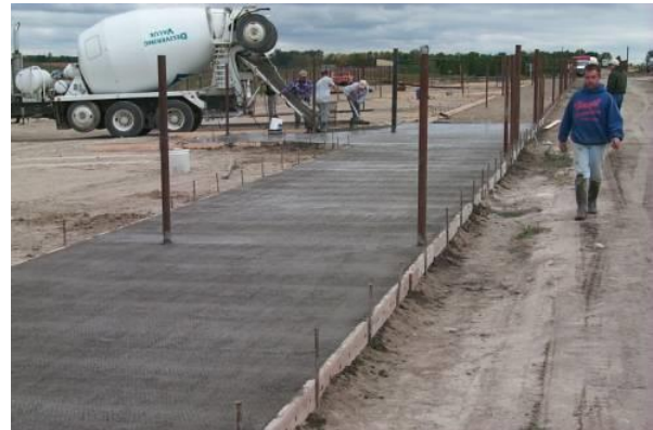
Figure 76. Construction of an apron using CLSM. Source: North Dakota State University
